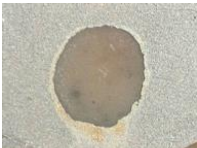
Electrode face at the point where lead wire separation occurred
